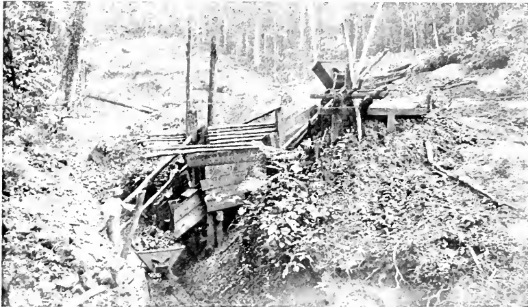
CHUTE BETWEEN FIRST AND SECOND LEVELS OF THE ORE-TRACK.
